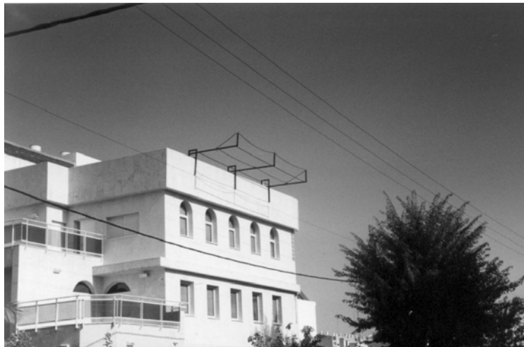
Figure 7: A house and a model of suppressing loop near a power line.
